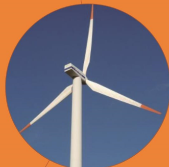
Wind power generation
